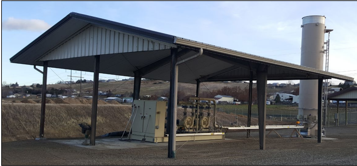
Exhibit 8. Flare Station Air Handling Skid and Stack
