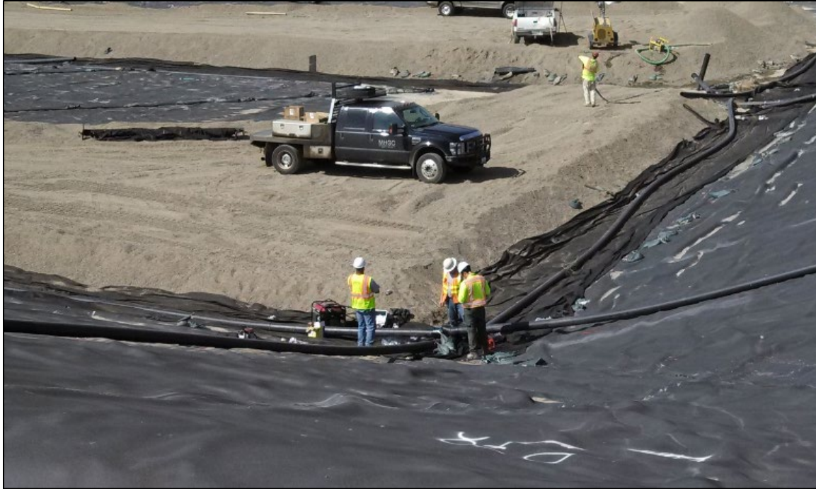
Exhibit 17. Cell D Construction Showing Sand Drainage Layer and Leachate Collection Pipes
